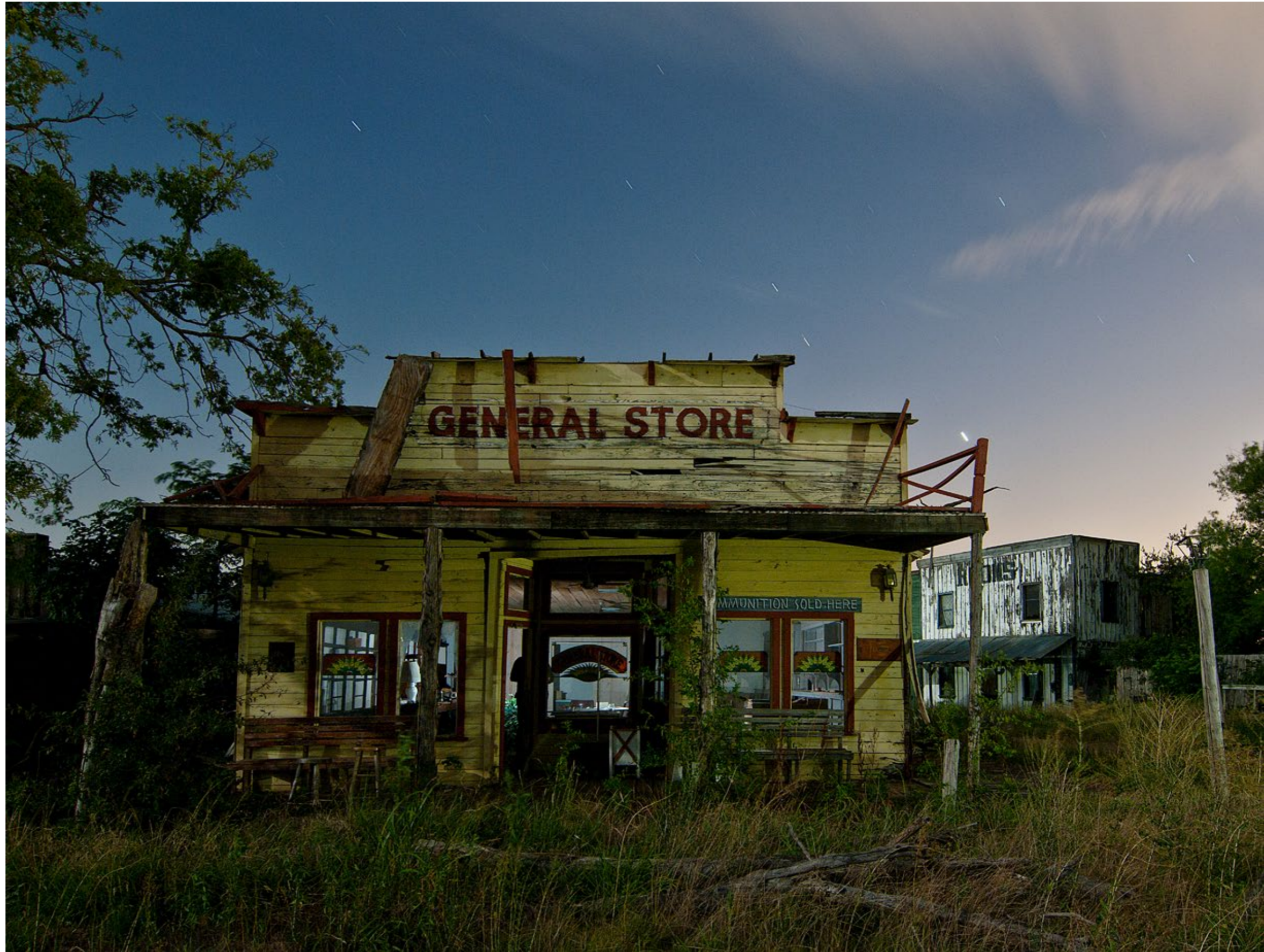
General Store – Abandoned old west tourist attraction, near Dallas, Texas, USA 2009. © Noel Kerns
